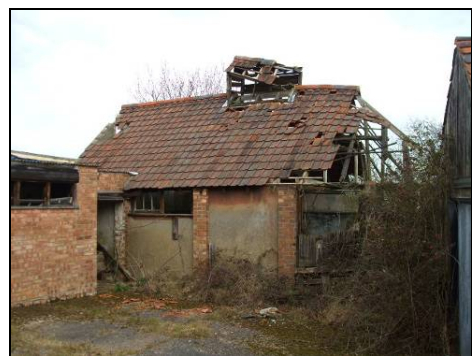
Farm buildings behind 'Gobions'
