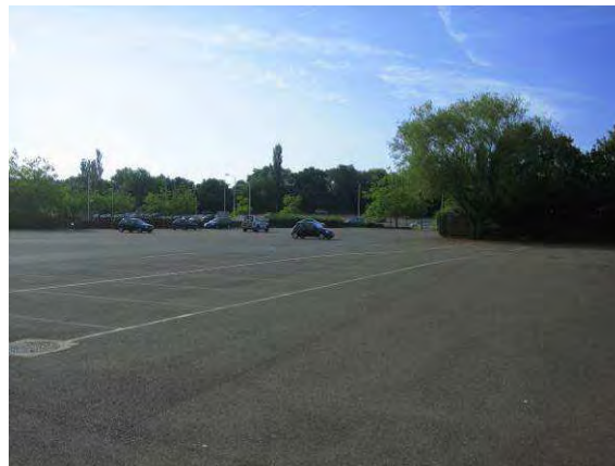
Plate 3 – Ashdon Way car park
