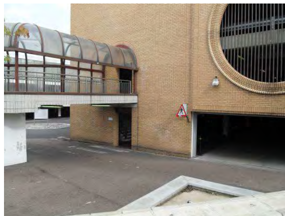
Plate 9 – Asda Multi-Storey Car Park access
