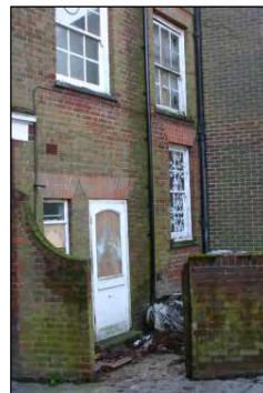
Rear of No.51a High St
