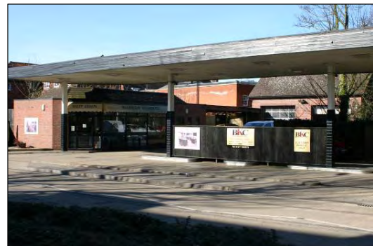
Former garage, Sun Street
