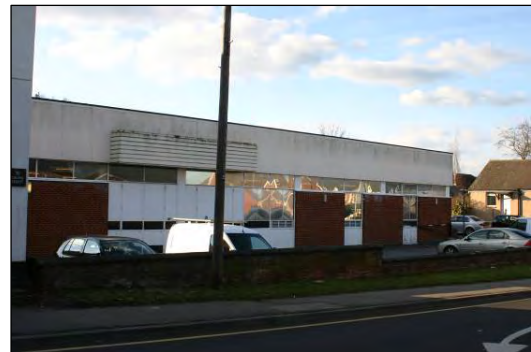
Telephone Exchange, Chapel Street
