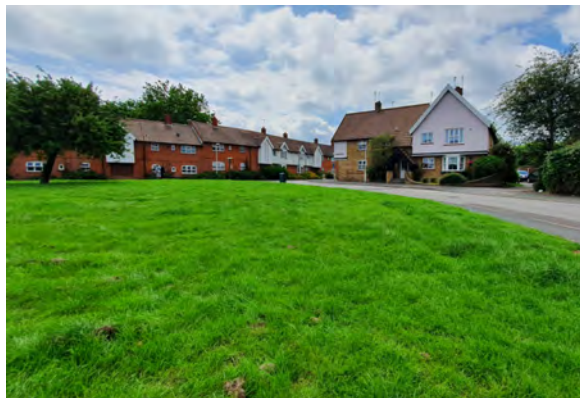
View 01: South towards Noak Bridge Village Green from Bridge Street -
