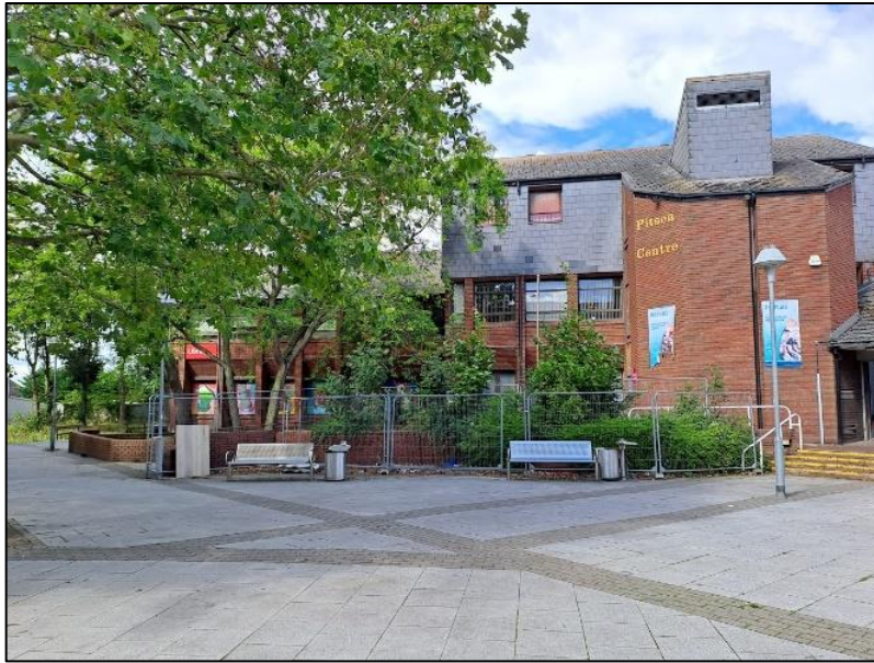
Figure 5.8: Pitsea Centre Building, Overgrowth and Fencing
