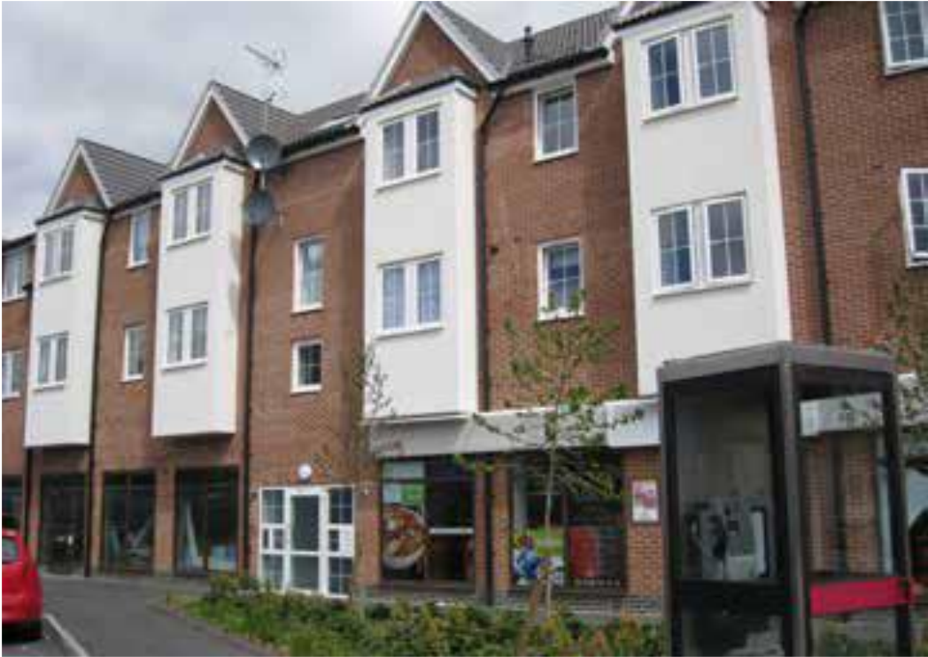
3.9 Beechwood Village Phase West is in construction:
