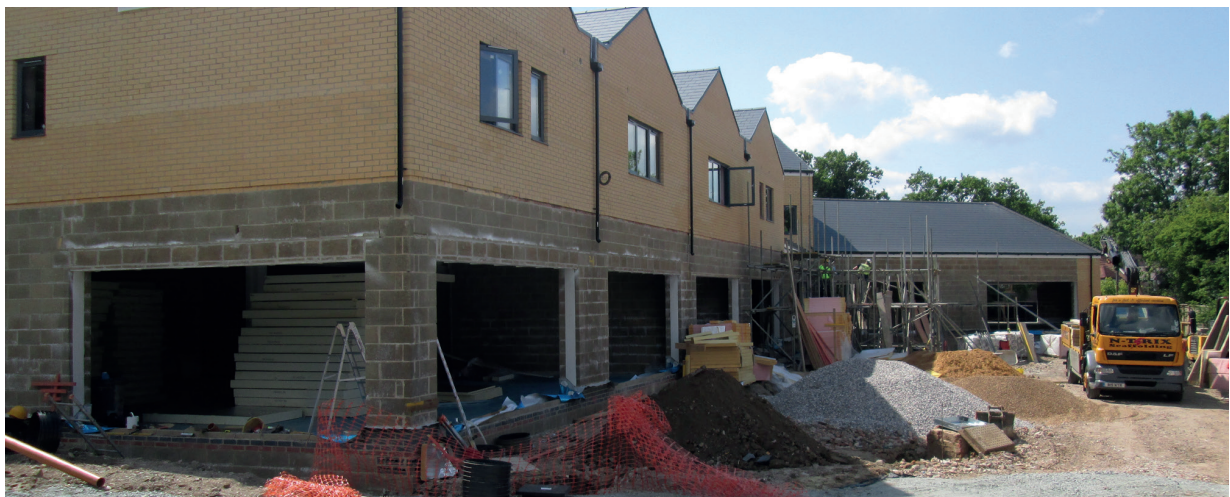
Lincewood Court, Langdon Hills
